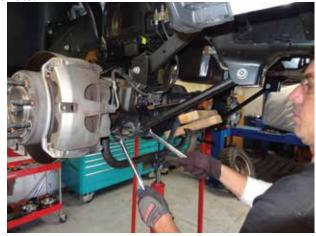
11. Use a die-grinder to completely cut-off the factory radius arm brackets from the factory frame. You are only cutting the weld, not the frame! DO NOT cut the factory frame. Do this for the driver & passenger side. If there is any excess weld left on the frame, grind it off so that the frame is smooth.
